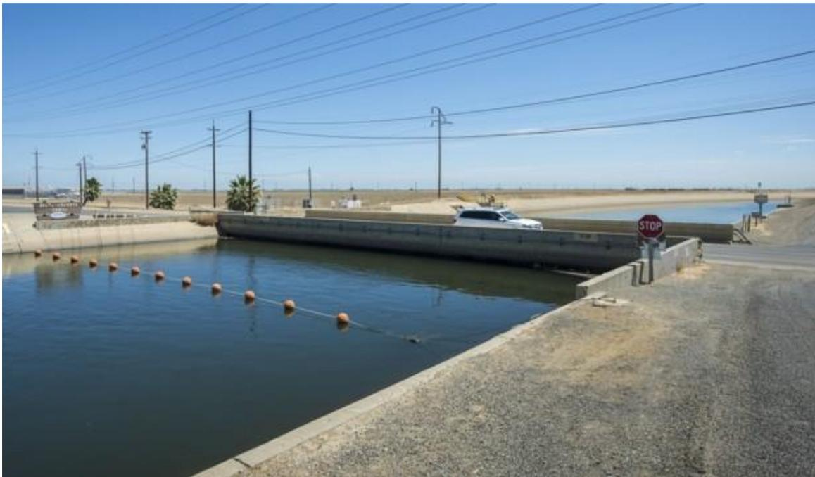
The drought has caused a bridge over a Firebaugh, California, irrigation canal to subside until there's almost no space between bottom of bridge decking and canal water surface. (Florence Low/ California Department of Water Resources via AP)
