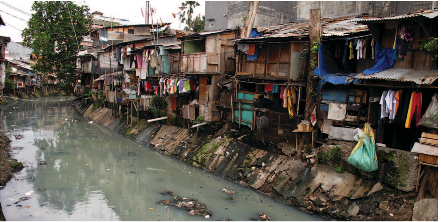
Rehabilitating Jakarta's waterways to mitigate flood risk. © Farhana Asnap/World Bank. Permission required for reuse.
